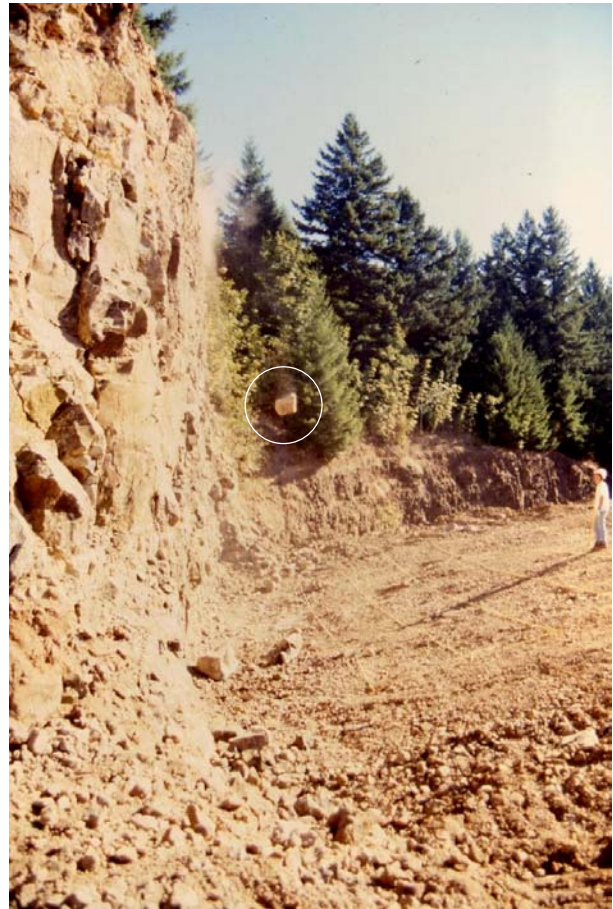
Figure 3.4: Rockfall testing; 40-foot high vertical presplit slope. Circle denotes test rock. Grid lines (middle-right) are for measuring impact and roll out distances.
