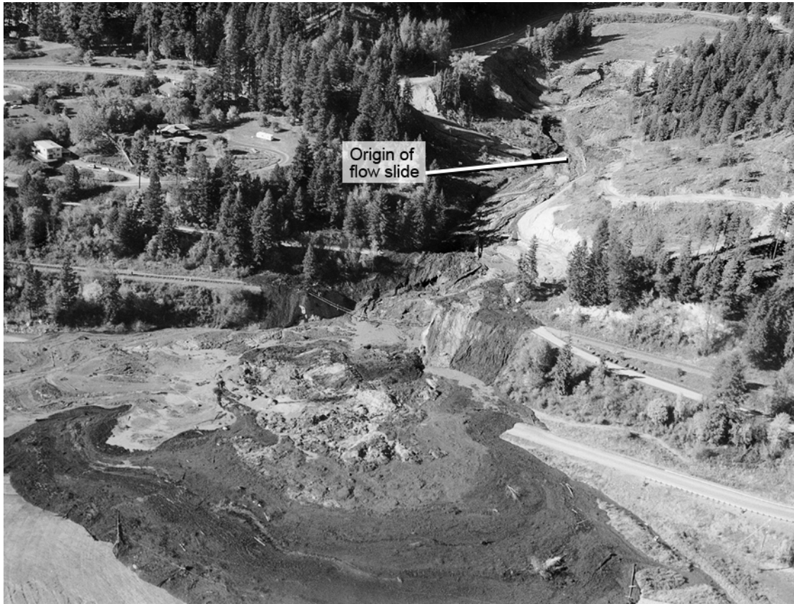
Figure 25. Bonners Ferry landslide. Aftermath of the major flow slide, showing rupture through the railroad embankment and into the flood plain (in foreground). (Photo: David Kramer)
