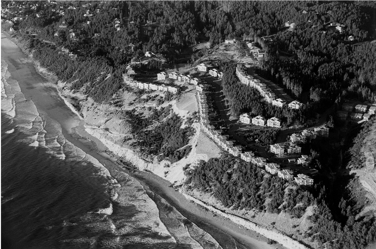
Figure 1. The Capes landslide. General view of slide adjoining the Pacific Ocean.
