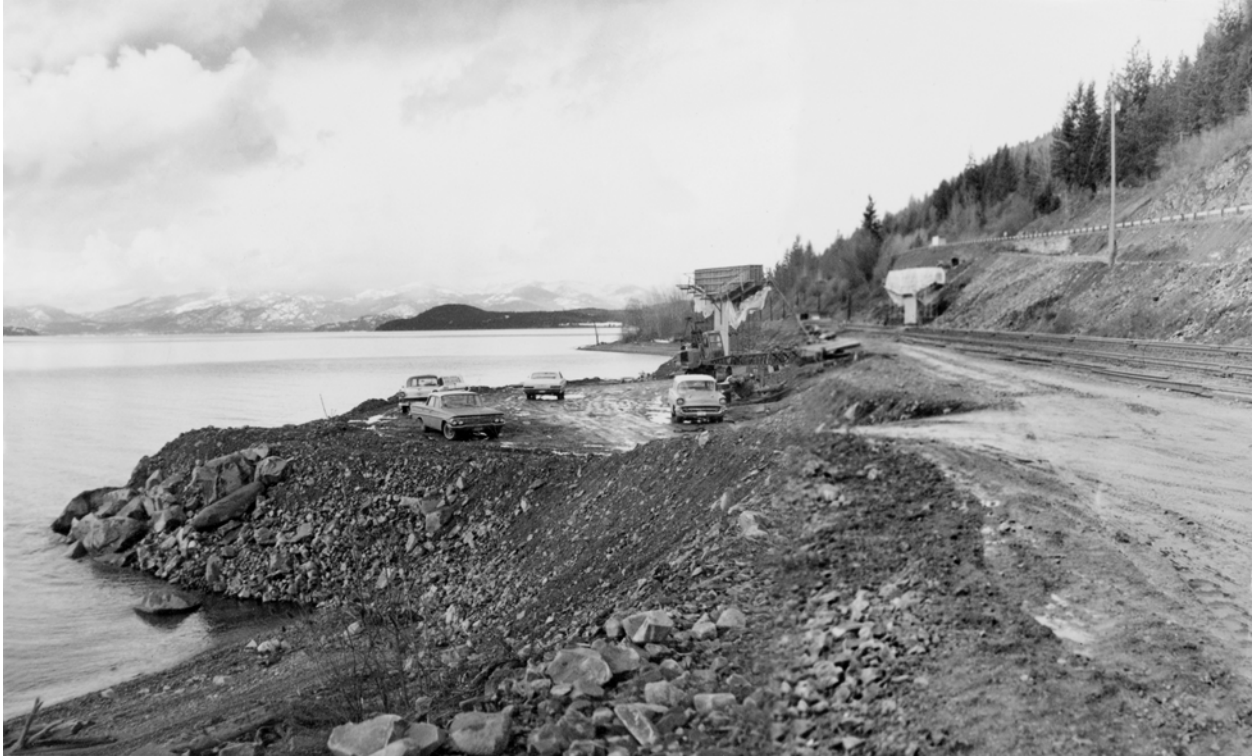
Figure 26. Lake Pend Oreille landslide. Hope Overpass site. Piers 2 and 3, on opposite sides of the Northern Pacific railroad tracks, are under construction in the background.
