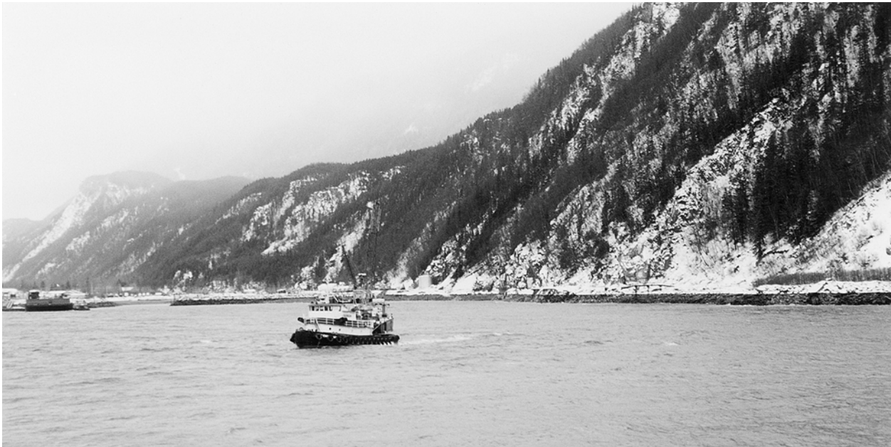
Figure 30. Steep rock walls on the east side of Skagway harbor.
