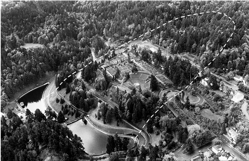
Figure 4. Washington Park Reservoirs landslide. The two reservoirs are at lower left. Perimeter of slide shown by broken white line.
