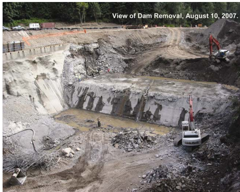
Figure 6. Dam Demolition in Progress
