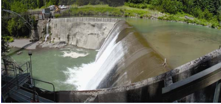
Figure 2. Photo of Marmot Dam
